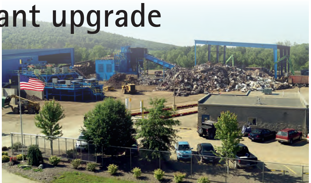
Upstate Shredding is investing US$ 25 million in a plant upgrade/expansion with the aim of making its Owego base one of the largest, most technologically-advanced and cost-efficient scrap metal processing facilities in the world.
