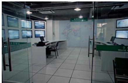
In WorldScrap's Global Monitoring Center, 16 large screens beam live images from scrap warehouses in Europe and North America to an operator, monitoring the loading of scrap metal at each location.
