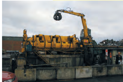
The company's new baling press from Italian manufacturer Colmar.
