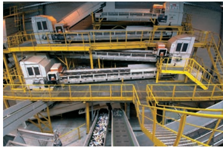
Waste treatment facility.
